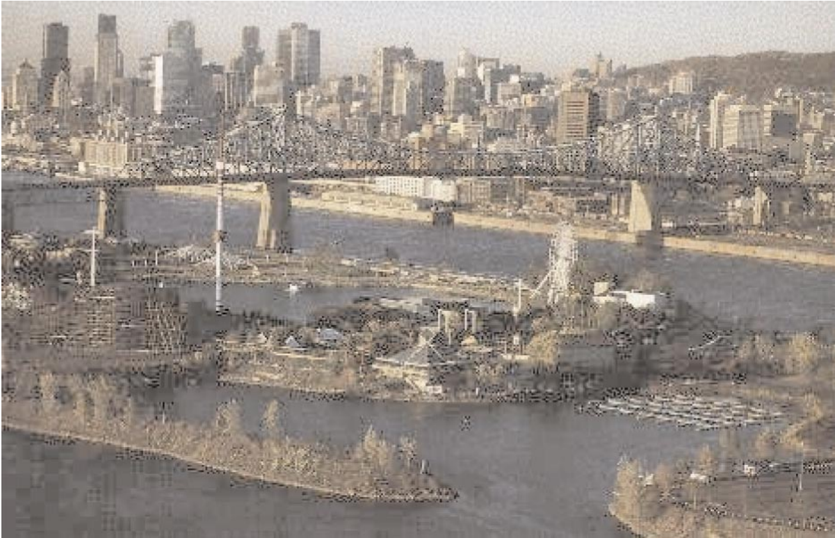
Montreal from NE—The Jacques Cartier Bridge and Downtown
