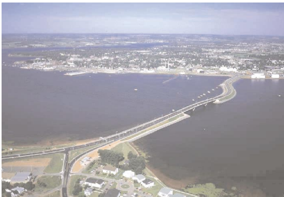
Charlottetown—The Hillsborough Bridge
