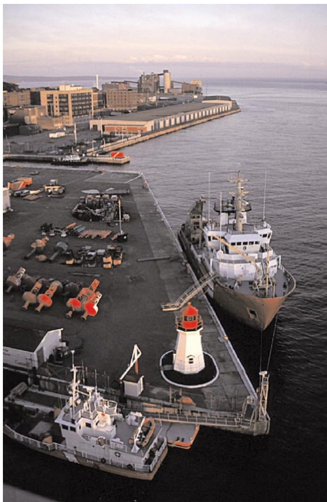
Saint John Harbor—Coast Guard Wharf (foreground) and Pugsley Wharf from N
