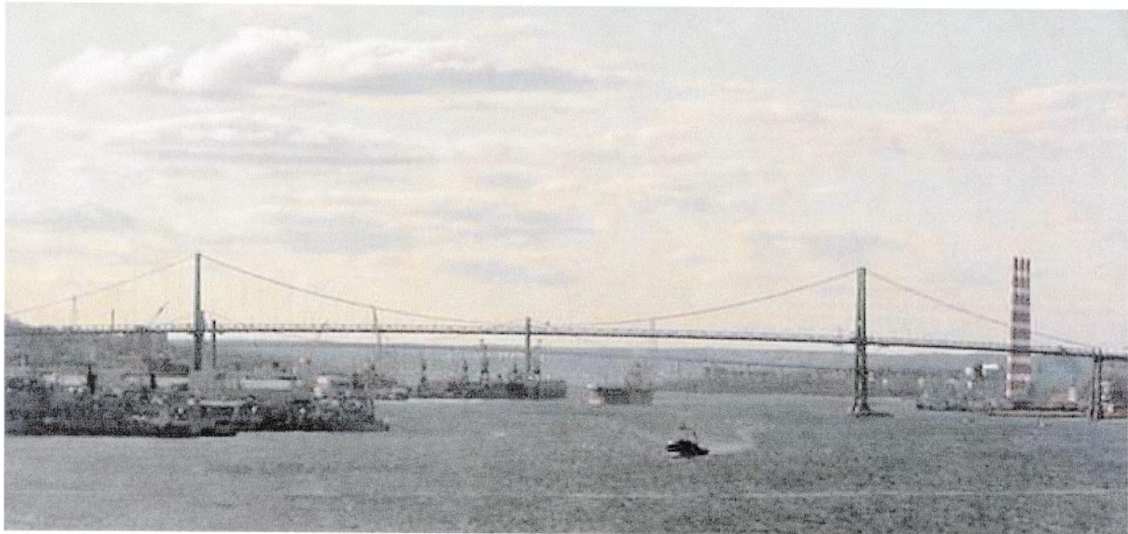
Courtesy of USCGC Healy Halifax Harbor—Macdonald Bridge (foreground) and MacKay Bridge (background)
