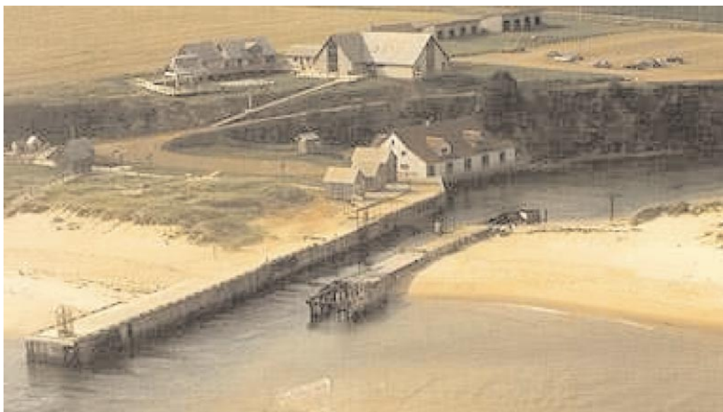
Souris—Basin Head Breakwater
